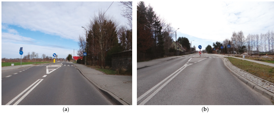
Figure 6. Test sections P9 and P10 in the village centre area: (a) P9—small lateral shift (1 m); (b) P10—big lateral shift (3 m).
