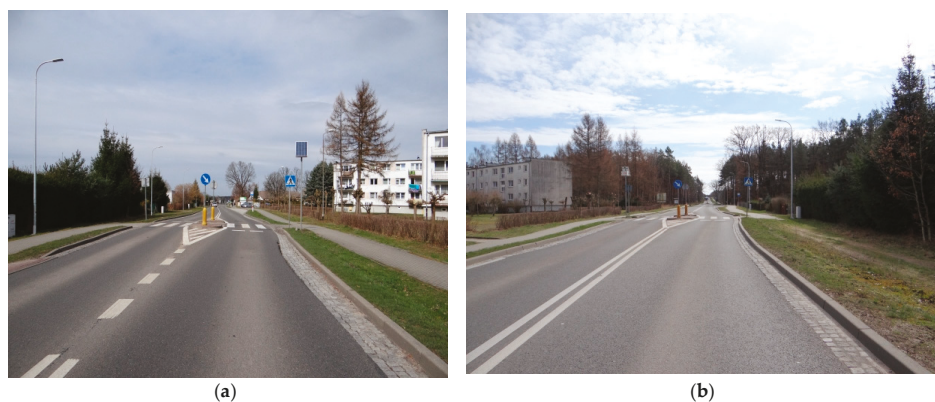
Figure 3. Test sections P3 and P4, pedestrian refuge placed 170 m after the gateway island symmetrical about the road centreline: (a) P3—exit zone; (b) P4—entry zone.
