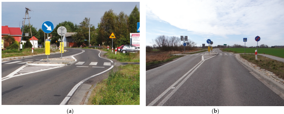
Figure 2. Test sections P1 and P2 with the pedestrian refuge positioned between the end of entry zone and beginning of the village centre area: (a) P1—entry zone; (b) P2—exit zone.
