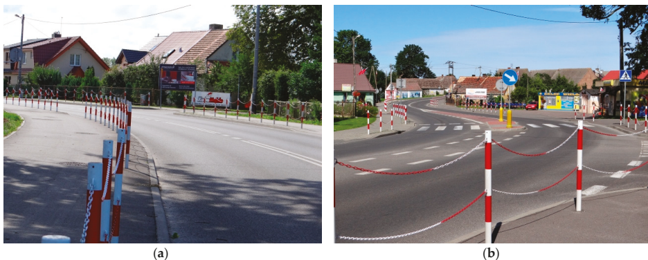
Figure 18. Stretch of the regional road lined with post-and-chain barriers: (a) in the village centre; (b) at the pedestrian crossing.
