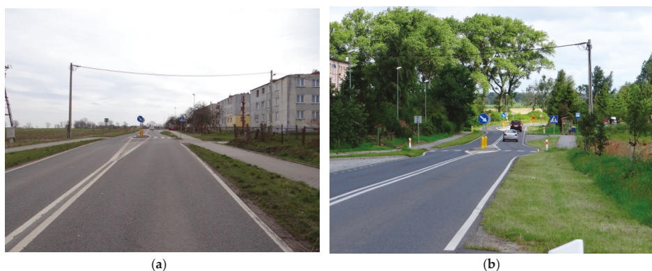
Figure 4. Test sections P5 and P6, pedestrian refuge placed 170 m after gateway island positioned on one side of the road centreline: (a) P5—entry zone; (b) P6—exit zone.
