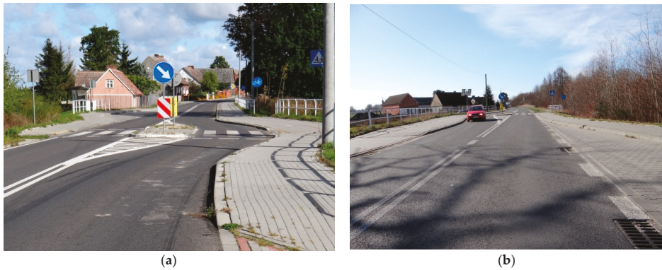
Figure 5. Test sections P7 and P8 between the end of entry zone and beginning of the village centre area: (a) P7—pedestrian refuge on one side of the centreline imposing large lateral shift by 2.5 m; (b) P8—departure lane without any imposed lateral shift.
