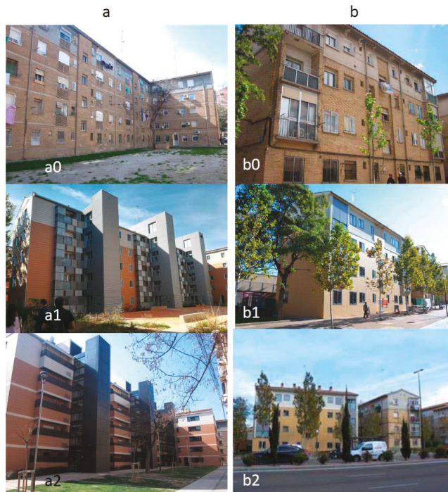
Figure 2. (a) Example of unity character loss after renovation with external insulation in Girón residential estate: (a0) original building image, (a1) example 1 of renovated building, (a2) example 2 of renovated building; (b) example of unity character continuation after renovation with external insulation in Alférez Rojas residential estate: (b0) original building image, (b1) example of renovated building, (b2) renovated building in context.
