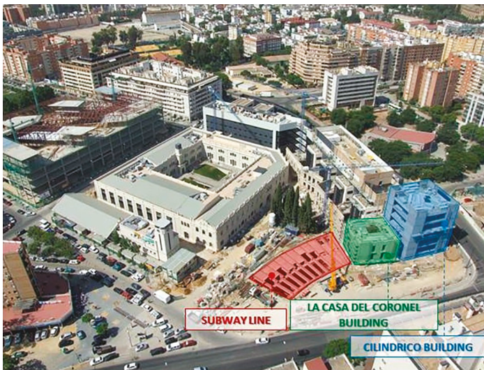
Figure 2. Execution of the works on the Cilíndrico and Casa del Coronel buildings over the Seville subway line. Source: The authors.
