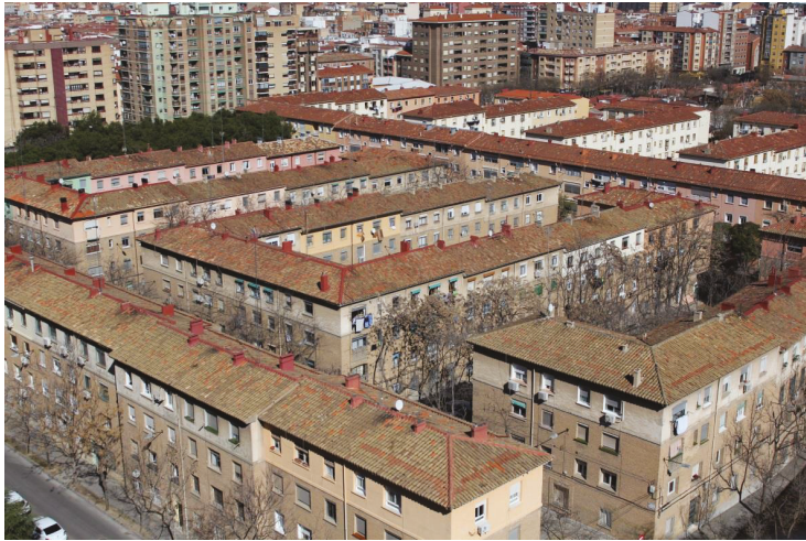
Figure 1. Example of social housing estate declared as urban area of interest (UAI) in Zaragoza: San Jorge.
