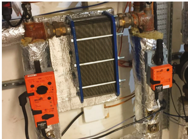
Figure 4. Small laboratory plate heat exchanger (PHX).
