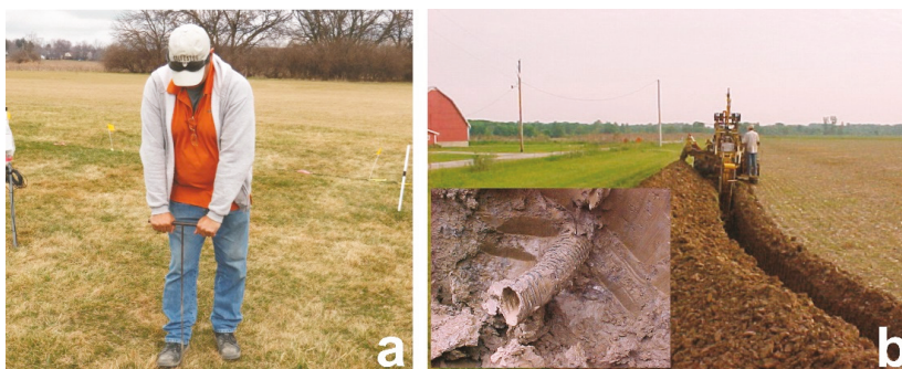
Figure 1. Present methods for finding drainage pipes: (a) hand-held tile probe; (b) heavy trenching equipment with inset photo showing an example of the drainage pipe damage caused during this excavation operation.
