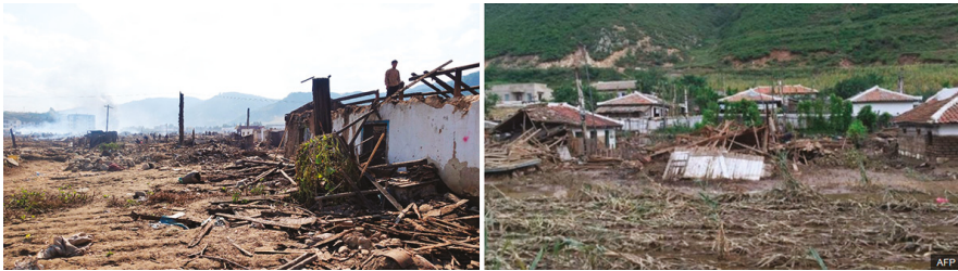
Figure 2. Flood damage in Hoeryeong City in August of 2016 ( http://kp.one.un.org/content/unct/dprk/en/home/emergency-response/floods-2016.html , http://www.bbc.com/news/world-asia-37335857 ).
