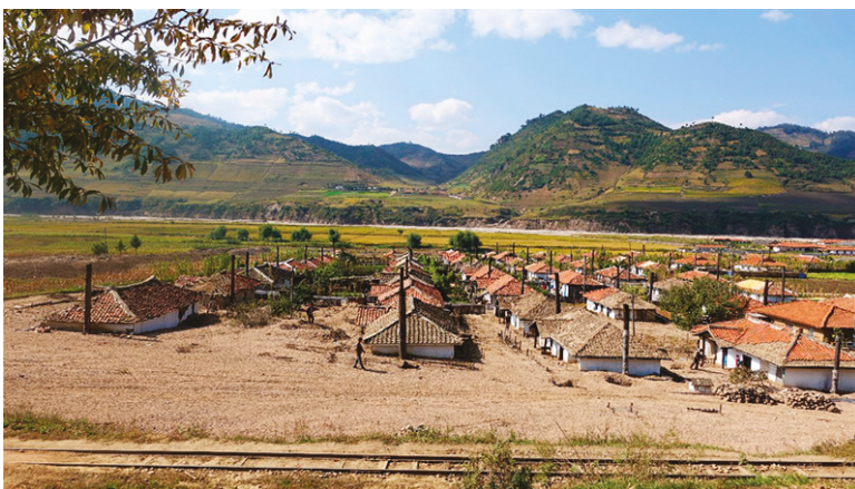
Figure 10. Flood-damaged residential houses in the study area (source: http://kp.one.un.org/content/unct/dprk/en/home/emergency-response/floods-2016.html ).
