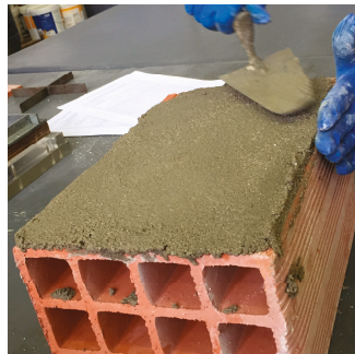
Figure 2. Mortar application on a brick.
