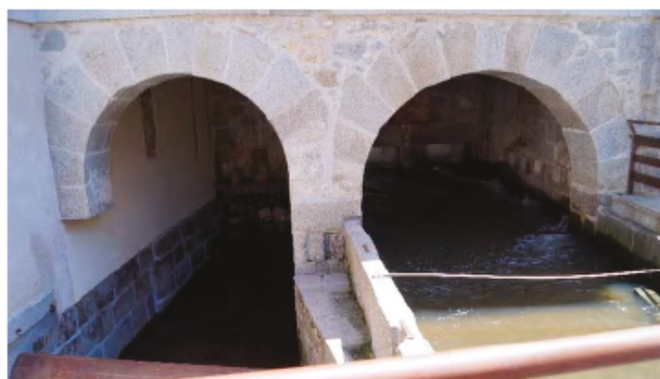
Figure 12. Entrance of the water flow in the SRMF. The right opening connects to the channel that feeds the waterwheels, while the left one returns the surplus water to the Eresma River. (Image property of the authors).
