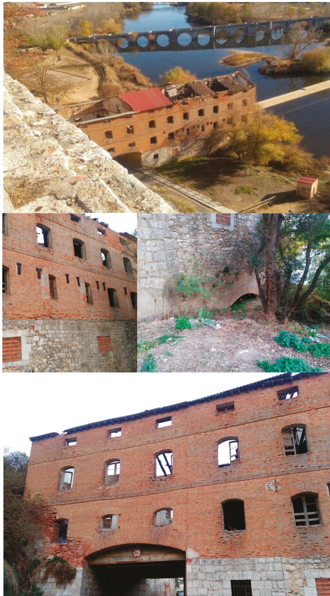
Figure 3. Photographs of the factory, 2019.
