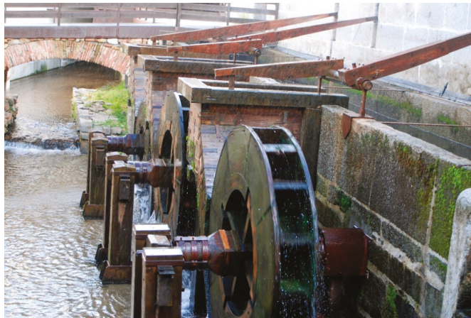
Figure 9. Forging shop waterwheels and the channels. (Image property of the authors).
