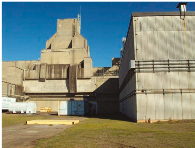
Figure 1. Reactor building 105-C at the Savannah River Site.
