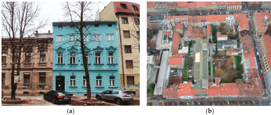
Figure 2. (a) Renovation of facades and energy upgrading of existing structures (b) Typical building blocks in Zagreb (photos by M. Stepinac).
