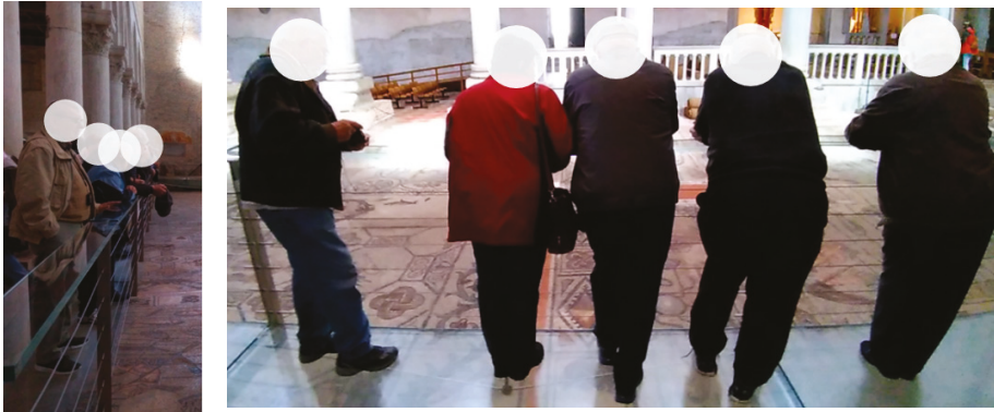
Figure 7. Example of service loads for the tested LG beams (photos by C. Bedon, courtesy of So.Co.Ba.).
