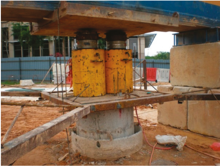
Figure 10. Existing platform in full-scale maintenance of the pile load test.
