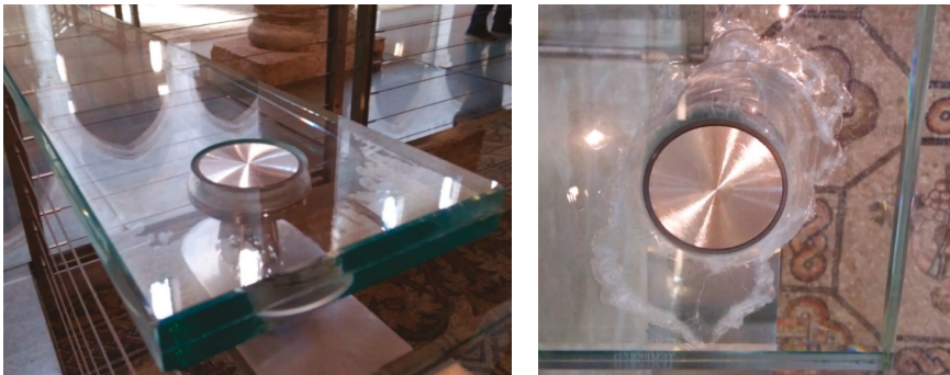
Figure 9. Example of delaminations (i.e., bubbles and shadows) for a selection of tested LG beams (photos by C. Bedon, courtesy of So.Co.Ba.).
