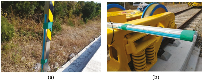
Figure 13. Simultaneous trigger system by a tape switch: (a) trigger for the high-speed cameras; (b) trigger for the data logger.
