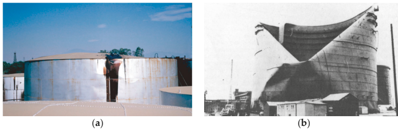
Figure 1. Failure cases of liquid storage tank. (a) Earthquake. (b) Wind [1].
