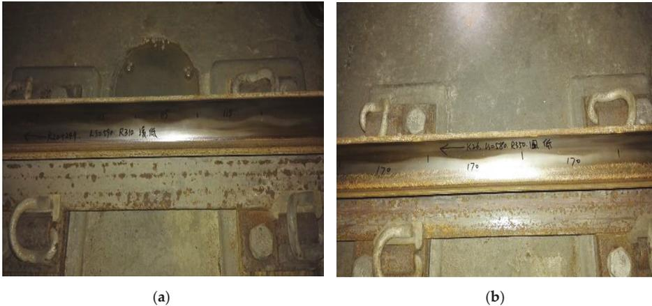
**Figure 16.** Rail corrugation in different sections: (a) section 1; (b) section 2.
