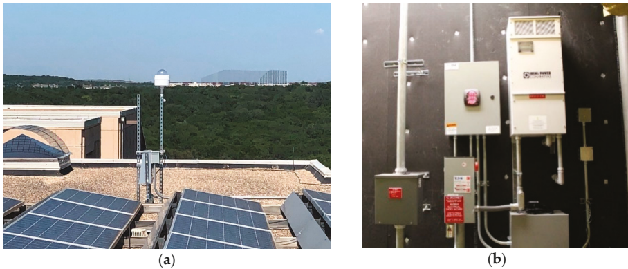
Figure 8. (a) PV panels and SkyImager at UTSA; (b) Inverters & combiners, Engineering Bldg.
