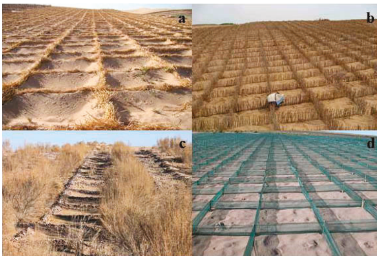
Figure 7. Various materials used for Checkerboards Barriers. (a) Straw; (b) Shrub branches; (c) Stones and Shrubs; (d) Plastic.
