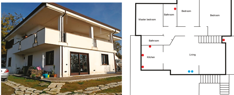
Figure 3. Case study building #3 with location of devices (red dots: smart-plugs, green dots: current clamp meters).
