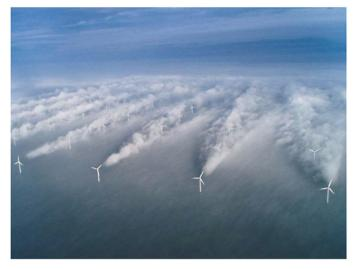
**Figure A1.** Image taken in February 2018 showing the obvious wake effects marked by humid air condensation in the Horns Rev OWF, Denmark.
