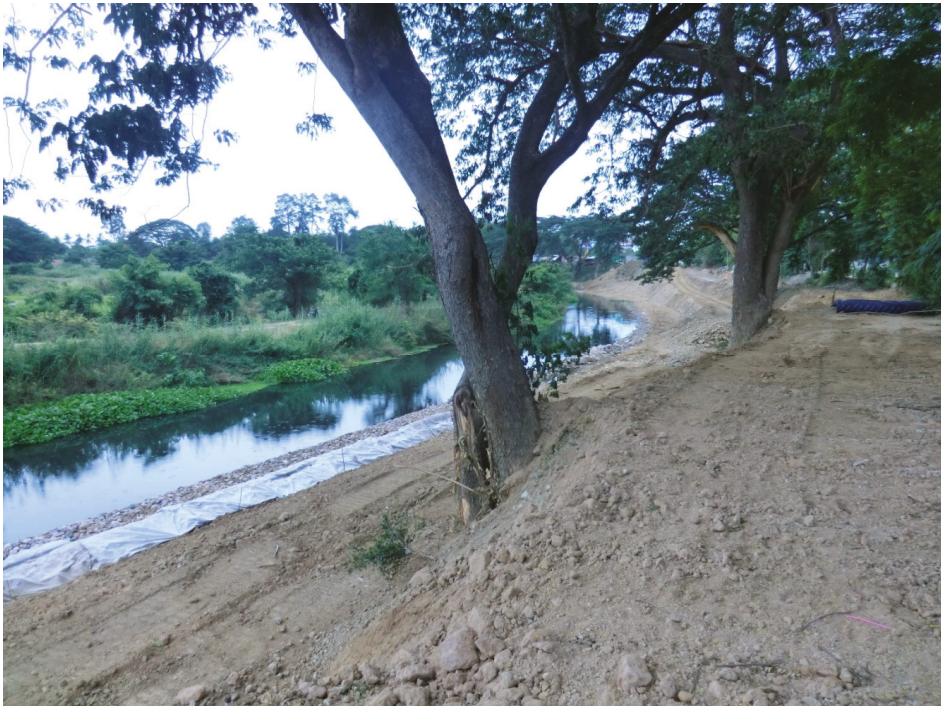
Figure 4. Channelization on a river system in the SIEP watershed. Photo by Jonathan Long.
