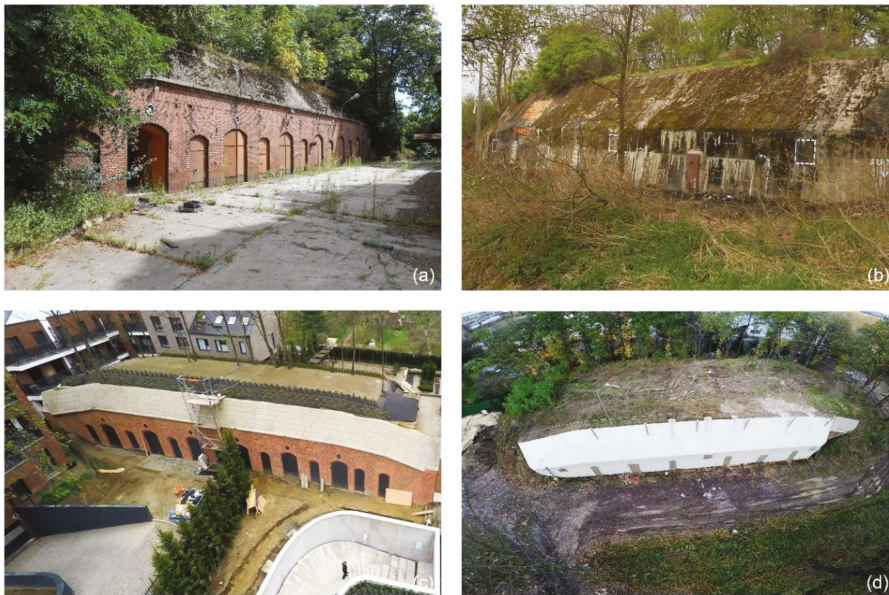
Figure 1. Examples of work that cause soil and plant ecosystem degradation of historical green roofs: (a,c) Infantry shelter before and after restoration; (b,d) infantry shelter before and during restoration works with a new green roof, Wrocław, Poland. 2012 and 2016, sourced from the author Lukasz Pardela’s archive.
