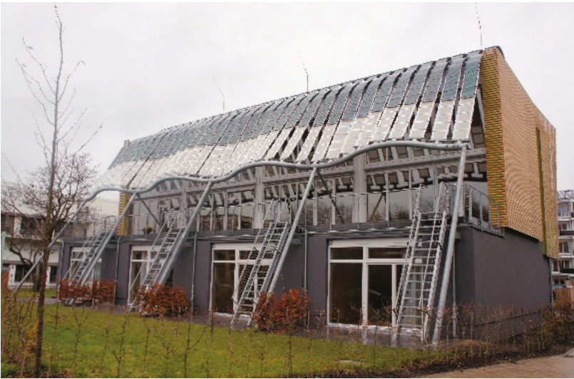
Figure 11. Solar electricity generating thin-film system independent of the building (photo by W. Celadyn).
