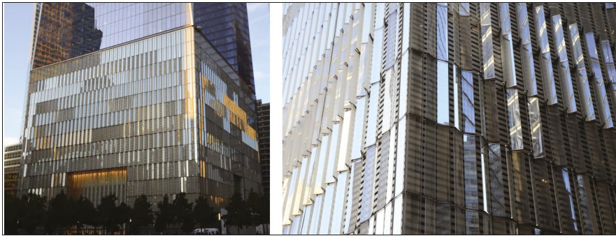
Figure 23. One World Trade Center: Reinforced concrete base with aluminum claddings and glass panels mounted in special profiles (photograph by authors).
