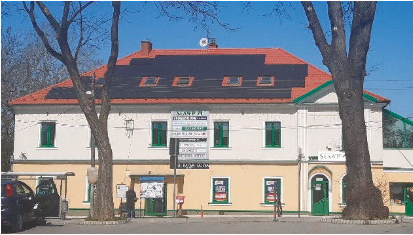
Figure 13. Disharmonious color composition on the building's roof covered with red ceramic tiles and monocrystalline PV panels (photo by W. Celadyn).
