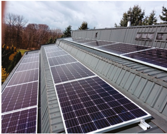
Figure 8. Stepped roof with PV monocrystalline photovoltaic panels installed at the recommended angle of 15°. Location: 49°57' N, 19°55' E (photo by W. Celadyn).
