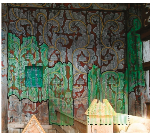
Figure 5. Example of mapping of conservation treatment in Kvernes stave church. The image shows the eastern part of the north wall in the nave of Kvernes stave church. Areas marked with green were consolidated with sturgeon glue (date: 5 April 2013). Photo © NIKU 2013.
