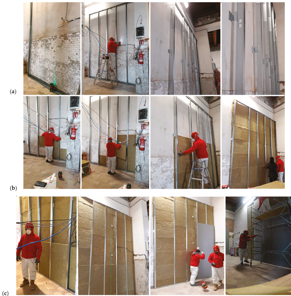
Figure 4. Installation of the selected insulation system.
