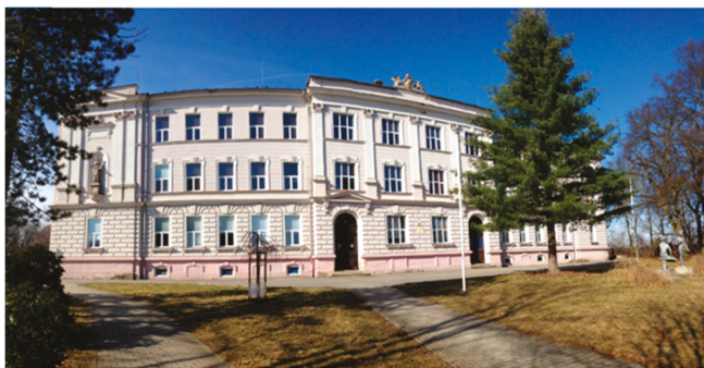
Figure 2. Historical building of primary school, locality Mimoň, CZ [37].
