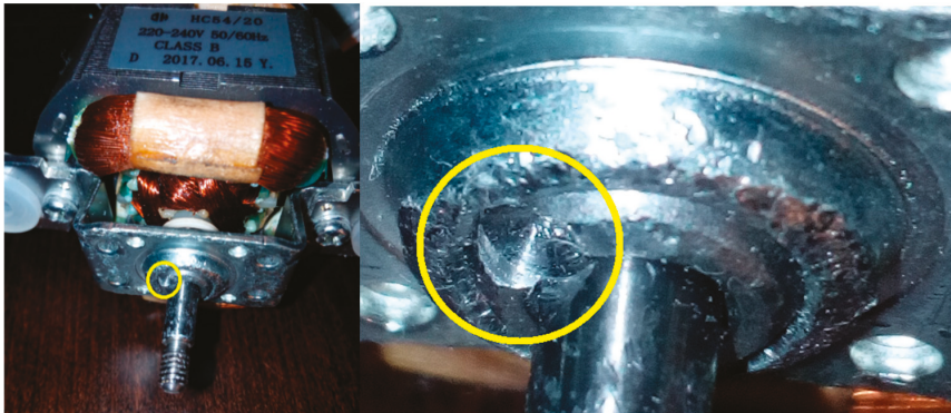
Figure 12. CG-B with a light damaged rear sliding bearing (indicated by yellow circle).
