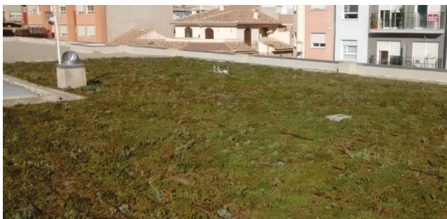
Figure 6. General view of greenroof.
