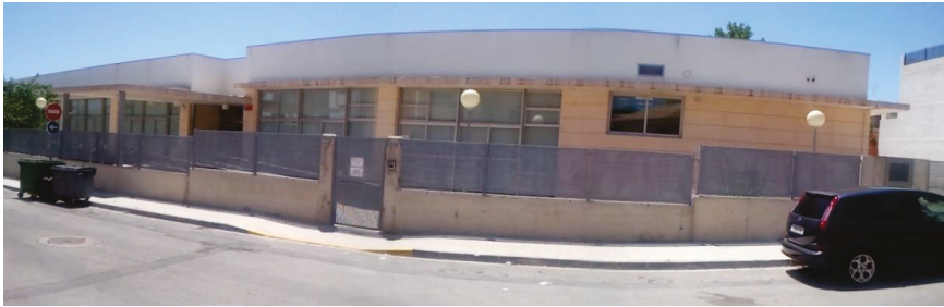
Figure 2. Building main facade (north).
