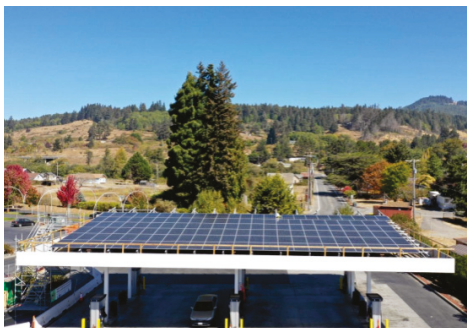
(a) 60 kW local solar power capacity
