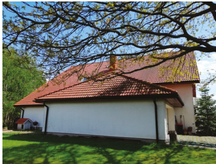
Figure 5. A view of the northern buffer space of the house.
