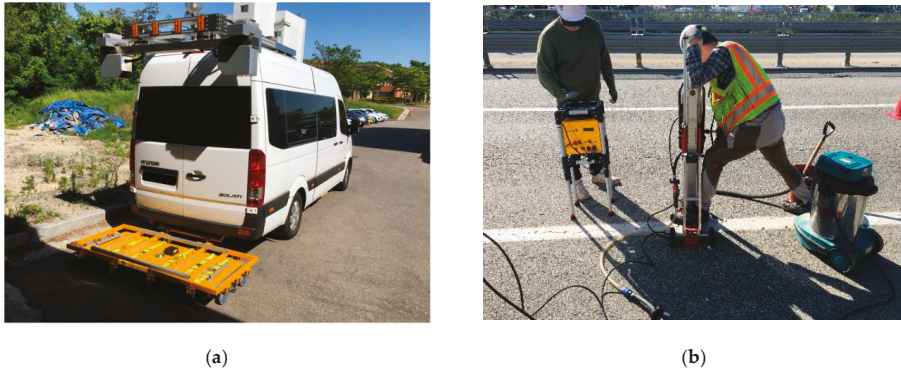
Figure 9. In-situ validation tests with (a) multi-channel GPR-mounted van and (b) core drilling.
