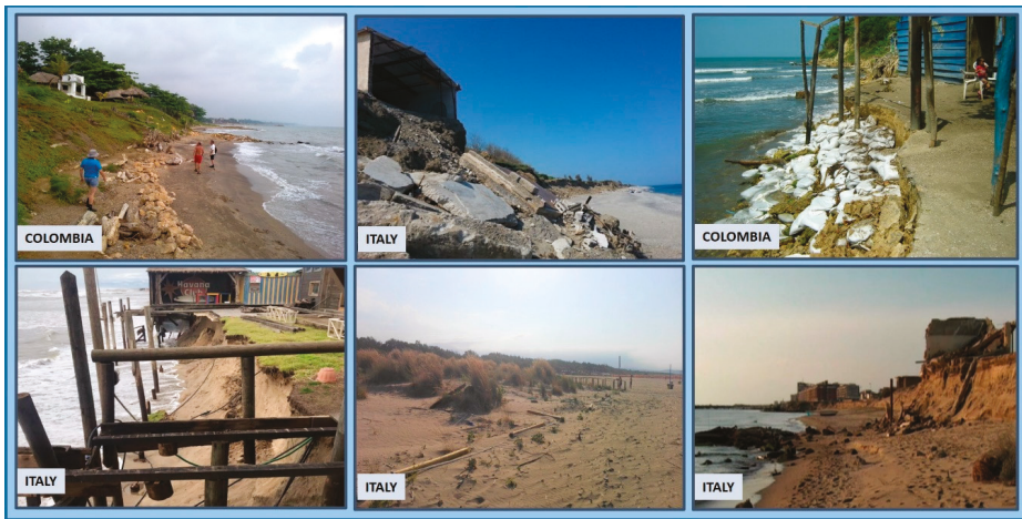
Figure 2. Examples of chronic erosion along low coastal areas in Italy and Colombia. Source: Giorgio Anfuso, Angela Rizzo, Gianluigi Di Paola.
