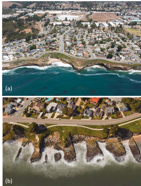
Figure 5. (a) Unprotected section of West Cliff Drive study area showing low eroding cliffs eroded into the Santa Cruz Mudstone [15], (b) oriented embayments eroded along parallel joints in the Santa Cruz Mudstone (Google Earth, 2018).
