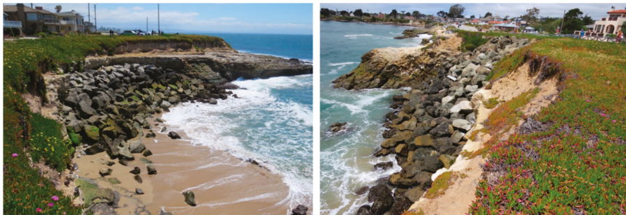
Figure 14. The placement of rip-rap over a 60 year period has reduced or eliminated bluff retreat along about 50% of West Cliff Drive, thus complicating any measurements of natural rates of bluff retreat.
