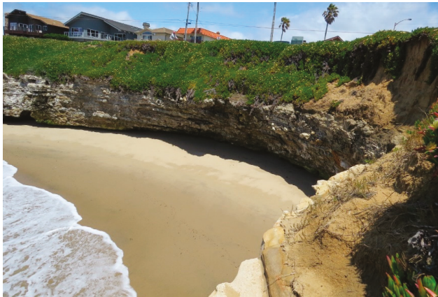
Figure 17. A section of coastal bluff consisting of the overlying weaker terrace deposits that are mostly vegetated, and the underlying Santa Cruz Mudstone that is being undercut. As in Figure 6, selecting the edge of the bluff for comparative measurements is difficult and somewhat subjective.
