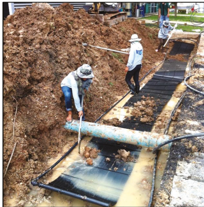
Figure 4. Carpet-type heat exchanger installation.
