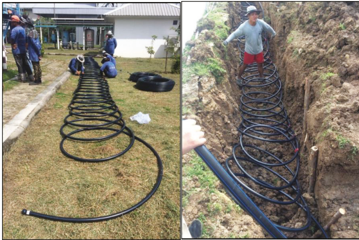
Figure 5. Installation of high-density polyethylene (HDPE) slinky pipes (Group 1).
