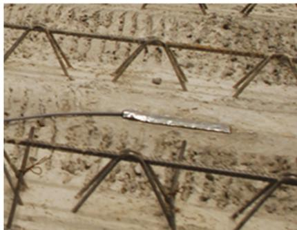
**Figure 1.** Fitting a strain gauge onto the surface of the lost formwork (reinforced concrete pre-slabs).
