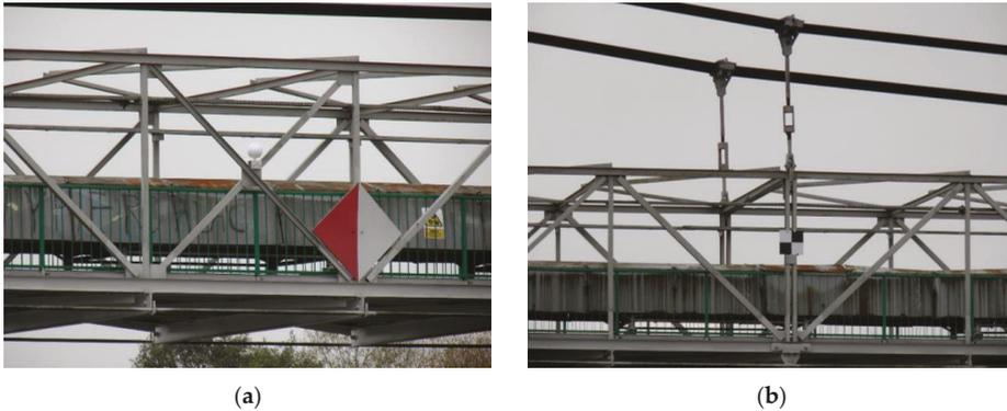
**Figure 7.** The supplementary measuring components fixed on the structure: (a) sphere, (b) measuring square shield (checker).
