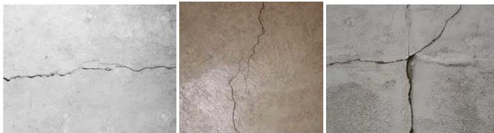
**Figure 5.** Example of images of concrete elements containing cracks.
