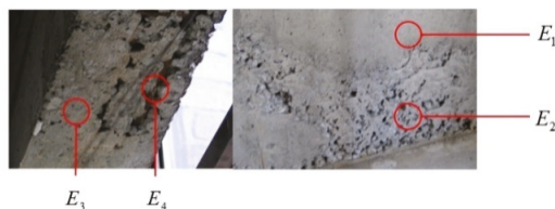
Figure 1. Different elastic modulus in different positions due to material heterogeneity.
