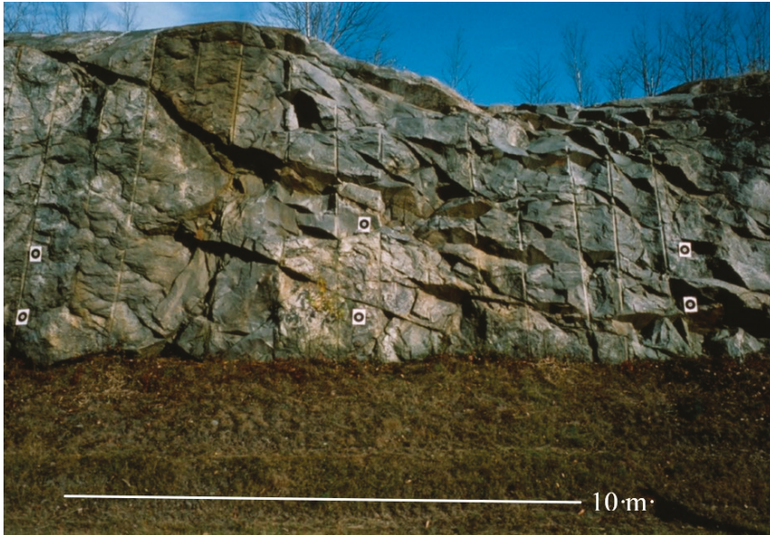
Figure 2. Photograph of a N5E striking roadcut exposure at the study site on I-93 containing NE striking, SE dipping faults included in this study. Note, most of the faults fractures exhibit dark planar surfaces. The rock type is primarily Concord granite (dark gray) with a Lower Rangeley schist block (light grey/white) exposed to the right of center above where the grass meets the bedrock and between the first and fourth drillhole from the left side of the photo. The subvertical lines are drill holes used in blasting the roadcut surface. Targets were used for rectification of photographs on which the geology and fractures were mapped by [16] (sheet 2).
