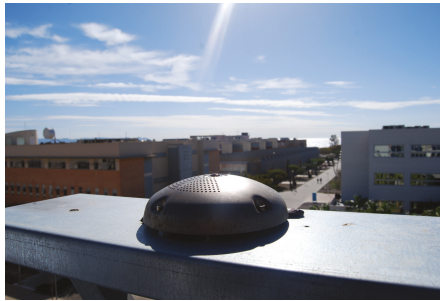
Figure 1. Mobotix Q24 camera installed in the University of Almería.
