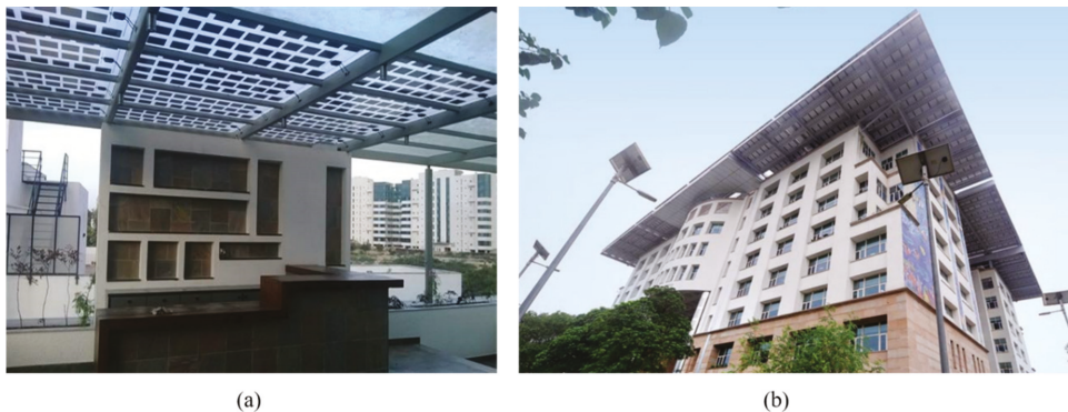
Figure 8. (a) Spaced type crystalline silicon solar-based BIPV roof for daylighting application (Source: HHV solar, Bangalore, India), (b) BAPV system in Indira Paryavaran Bhawan India (Image source: BT).
