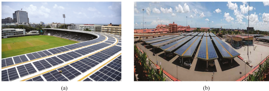
Figure 7. (a) World's largest solar rooftop with a capacity of 820.8 kWp installed on Braboune stadium, at Cricket Club of India, in Mumbai (18.93° N, 72.82° E) (b) India's largest solar carport 2.67 Mw at Cochin International Airport (Cial) (10.15° N, 76.39° E).
