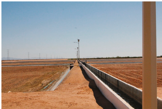
Figure 3. Infiltration basins in San Luis Río Colorado, Sonora, when empty.
