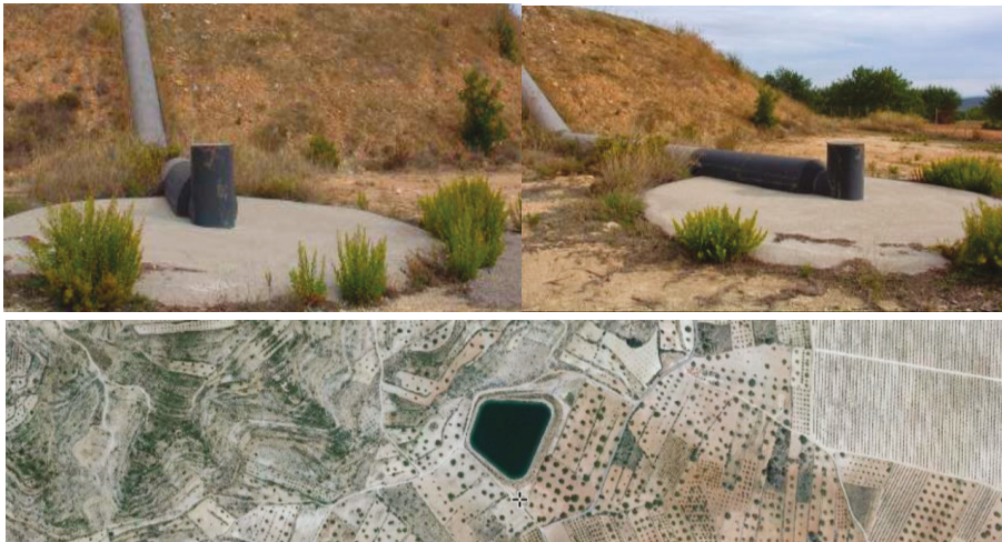
Figure 9. Deep borehole “Arnachos” at Balsa del Campo, Valencia (UTM 685,744/4,391,256) located in the margin of an irrigation pond and used as both, a safety and recharge element. Photos courtesy of J.M. Montes and FEGA.
