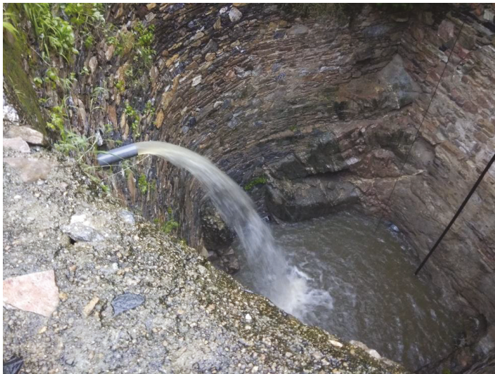
Figure 3. Runoff discharge into well after it was collected in the pit and had passed through the filter.
