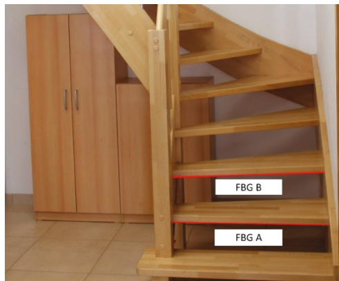
Figure 4. Placement of FBG sensors on the staircase in the smart home (SH), room R104.
