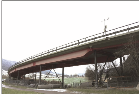
Figure 10. Crêt de l'Anneau Bridge near Neuchâtel (Switzerland).
