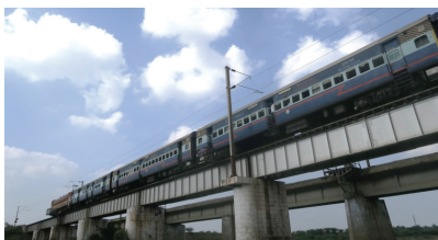
(a) System of bridges over the Arani river
