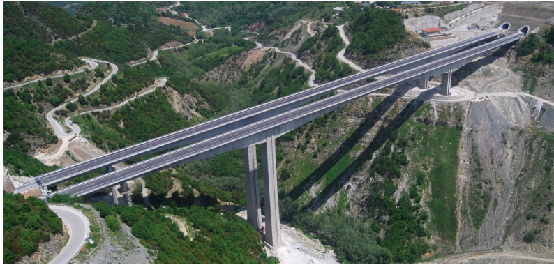
Figure 1. Picture of the Metsovo bridge.
