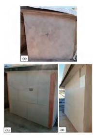
Figure 2. Selected test rooms in their original state (a) and during aerogel panel installation (b,c).
