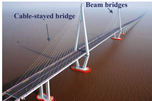
Figure 1. Overview of the cable-stayed bridge and beam bridges.
