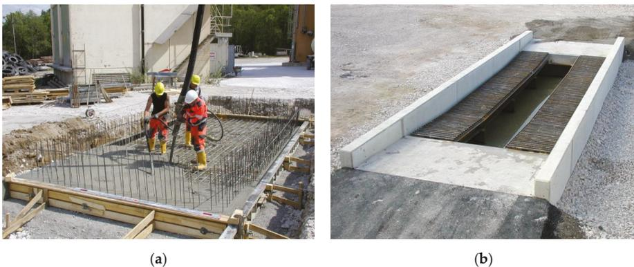
**Figure 11.** Test track construction using (1) CEM V/A (S-V) 32.5 R using a cement content of 400 kg/m<sup>3</sup> and a water-binder ratio of 0.45 during (a) concreting work and (b) after finishing the construction.
