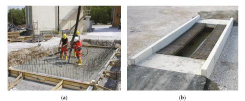
Figure 11. Test track construction using (1) CEM V/A (S-V) 32.5 R using a cement content of  $400 \text{ kg/m}^3$  and a water-binder ratio of 0.45 during (a) concreting work and (b) after finishing the construction.
