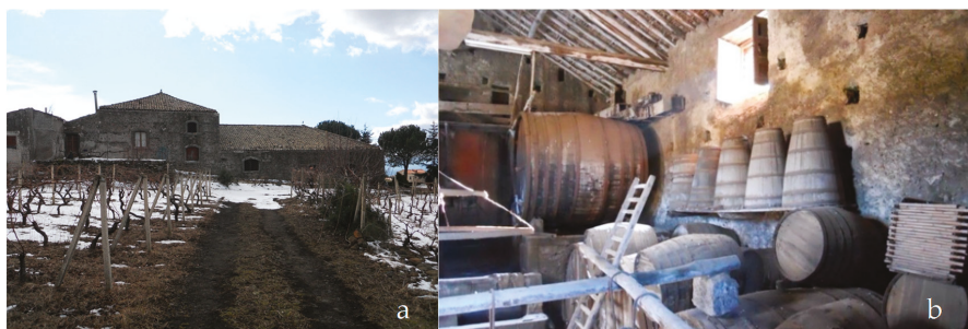
Figure 1. (a) The north façade of the wine cellar; (b) internal room of the wine cellar.
