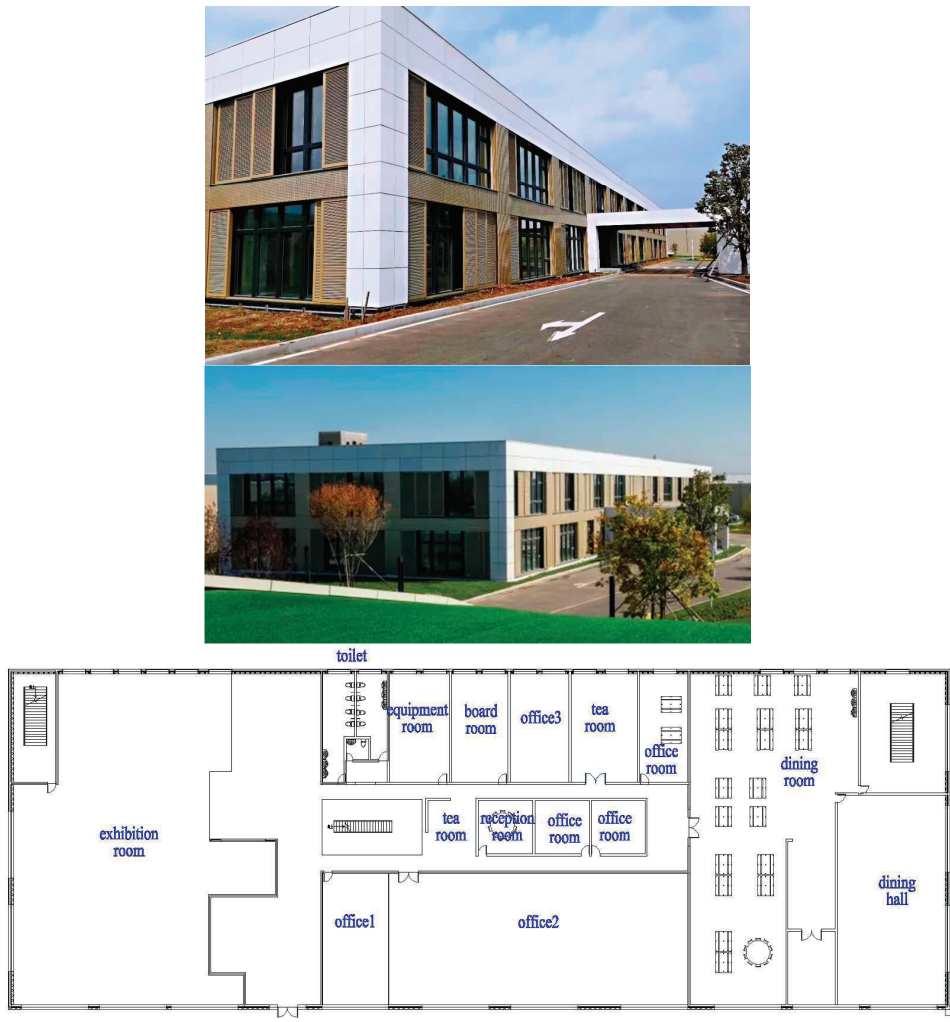
Figure 1. Senying passive office building: close and panoramic photographs (upper and middle panels), and ichnography of the first floor (bottom panel).
