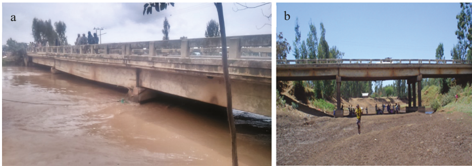
Figure 1. Gumara river at the bridge in the Fogera plain where the road from Bahir Dar to Gondar crosses; (a) August 2017 at flood stage during the rain phase and (b) February 2015 during the dry season when the flow has ceased (courtesy: M. M. Moges).
