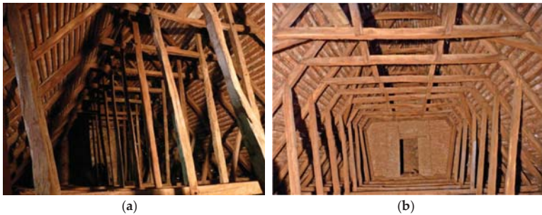
Figure 2. Romanesque roof structures: (a) roof structure Lutheran church in Vurpar; (b) roof structure Lutheran church in Toarcla.
