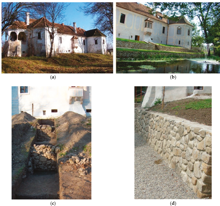
Figure 12. The castle facade towards the pond with the retaining walls in 2014 (a) and after the reconstruction in 2016 (b). The archaeological excavation of the retaining wall (c) and the renewed retaining wall (d). Photos by Fekete, A, 2017.
