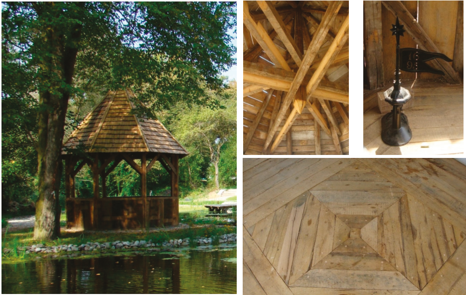
Figure 13. View and technical details of the gazebo in Miklósvár, constructed according to historical descriptions and analogical examples and used as an eye-catcher. Photo by Fekete, A., 2017.
