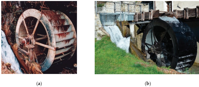
Figure 5. The overshot water wheels of the Riviera mill: (a) Before the renovation (Courtesy of Arch. Roberto Olivero, 2004); (b) after the renovation.
