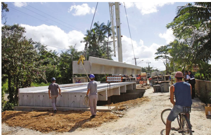
Figure 18. Obstacle transposition kit over Motucas River, at Estrada dos Portugueses, Vila Nova neighborhood, Joinville-SC - Type P23 PMD 5V. Source: Joinville City Hall [75].
