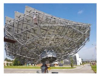
Figure 10. Installed solar concentrator in its working position.
