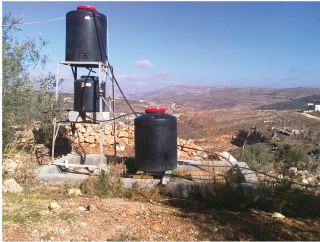
Figure 1. Onsite grey water treatment plant, Duara Al Qare'-Ramallah.
