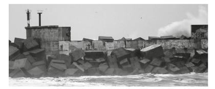
Figure 18. Displacement of the upper part of the crown wall in the breakwater of A Garda, Spain (2017).
