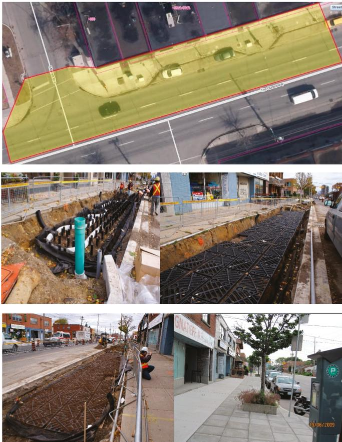
Figure 2. Construction phases of the Toronto underground RBR without a surface layer.
