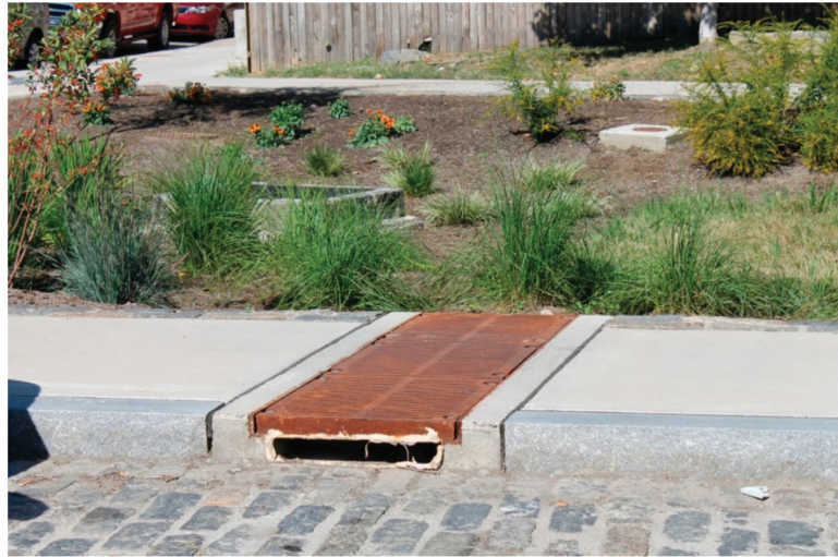
Figure 3. Rain garden in a former parking area in a residential neighborhood in Philadelphia (PA).
