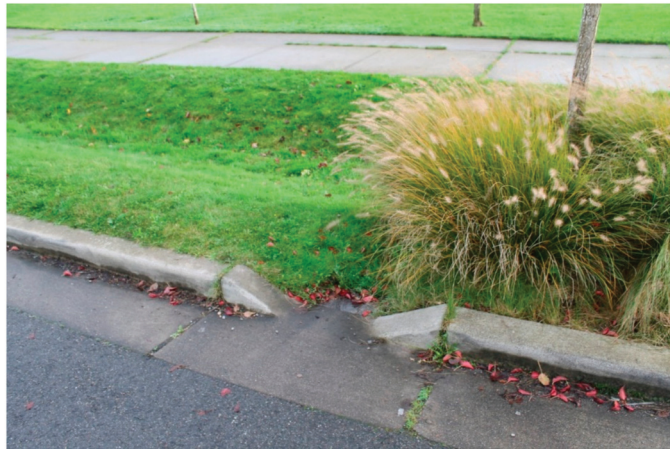
Figure 1. Green strip in Seattle (WA). The curb is lowered to allow runoff to infiltrate through a green trench.
