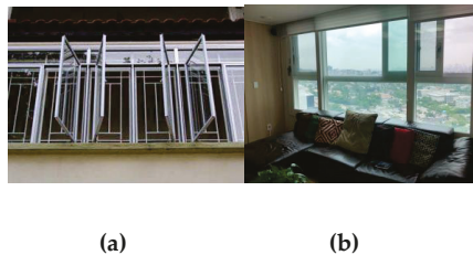
Figure 9. Window types: (a) Singapore (single-layer), (b) Korea (double-layer).
