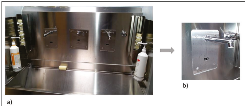
Figure 3. SHWOs with sensor-activated faucets and TMVs (a) and a sensor-activated faucet (b).
