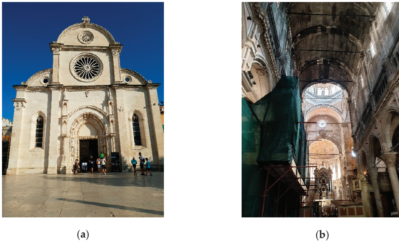
Figure 6. Cathedral of St. James in Šibenik, Croatia. (a) West view of cathedral and (b) iron tie rods inside the cathedral.
