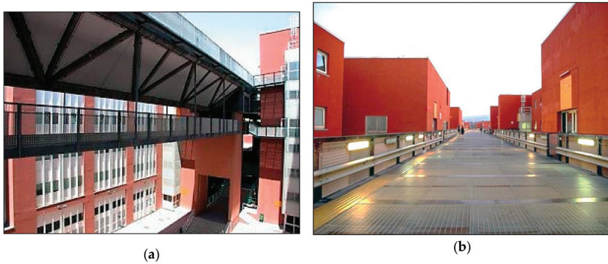
Figure 3. The bridge at the University of Calabria: (a) the pedestrian deck; (b) the upper deck.
