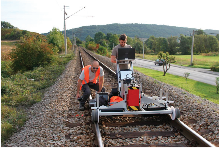
Figure 6. Conduction of GPR investigations.
