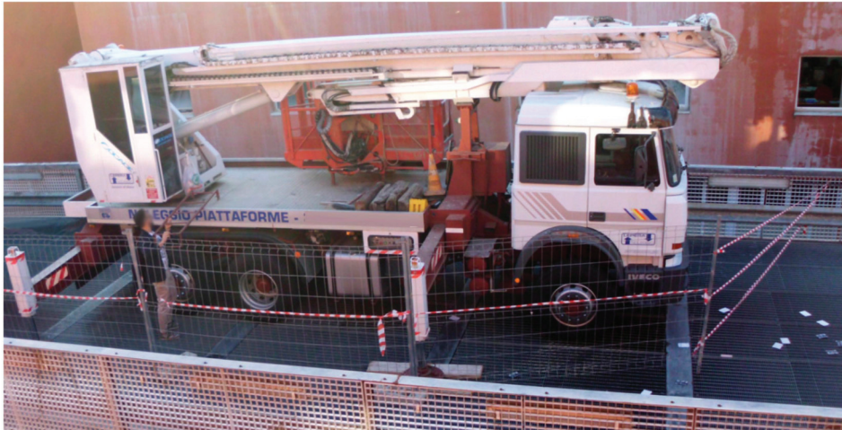
Figure 6. The truck elevator, used as static load.
