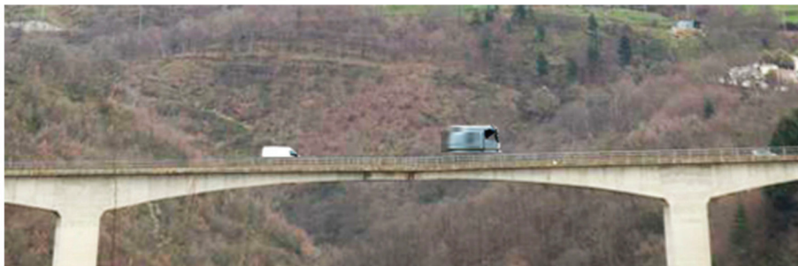
Figure 13. A frame of the video used to obtain position and estimate of the mobile loads.
