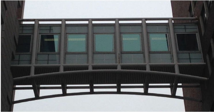
Figure 2. Mudd Schapiro Link Bridge.
