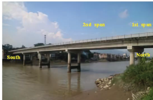
(a) Photo of Lieshihe River Bridge
